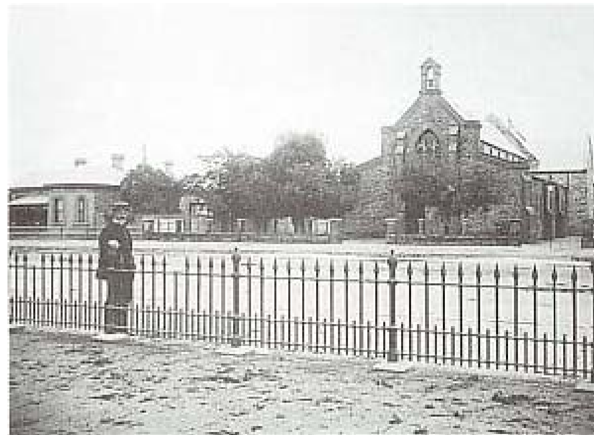
Figure Photograph of St Luke’s Church in c.1890s as published in The Heritage of the City of Adelaide (1990) by Marsden et al p. 197. Note the cast iron palisade fencing around the Square with each post set on a stone foundation stone. Source: ACC Archives.
